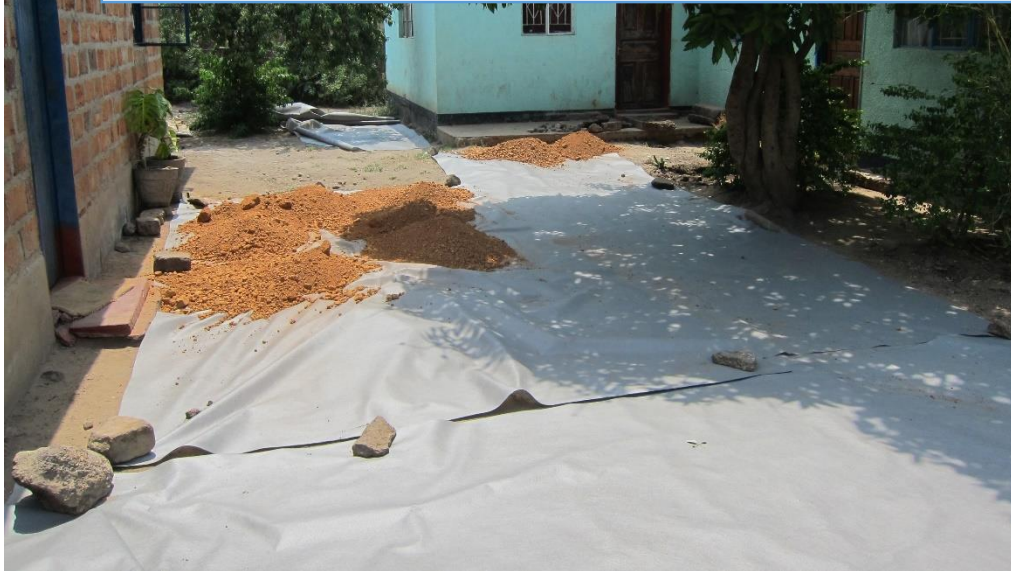
Laying Water permeability sheets around houses
